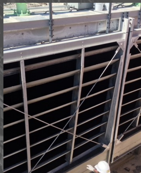
BAC Fluid Cooler Coil Replacement
